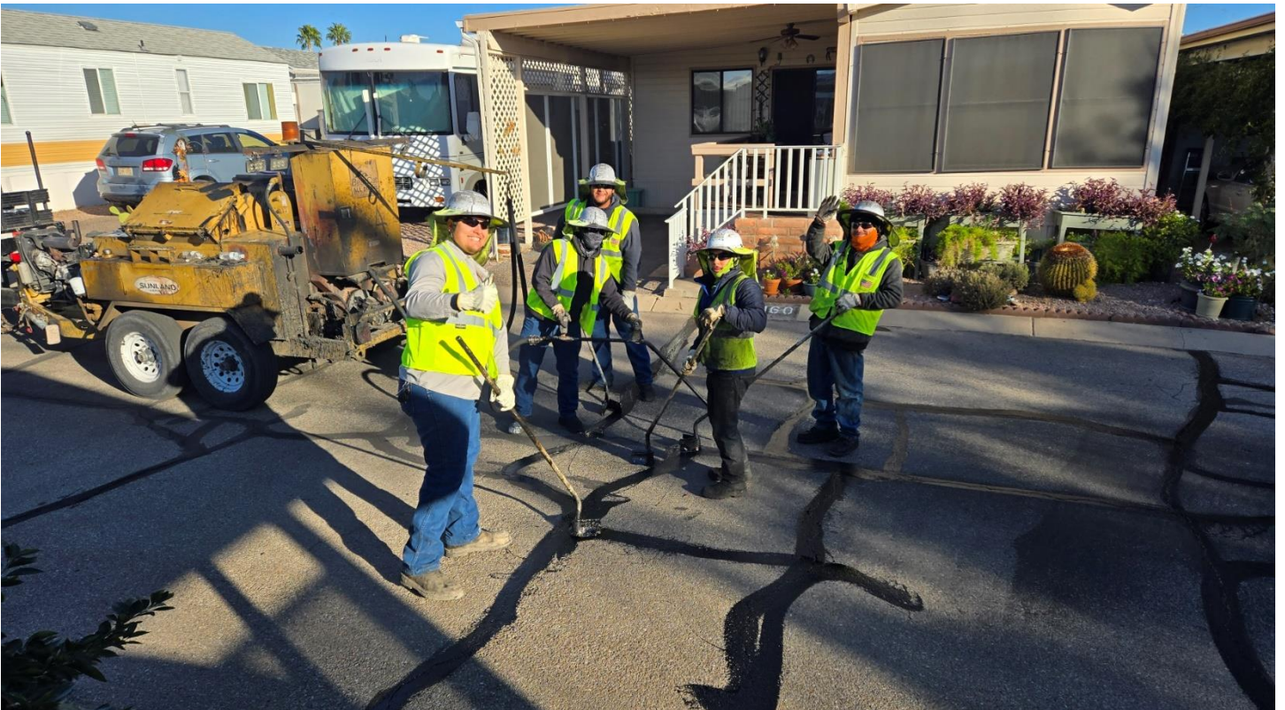
CRACK SEAL – photo compliments of Sally Van Atta
