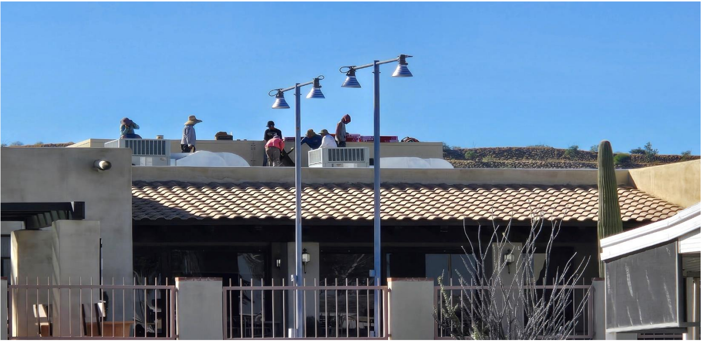
ROOF REPAIR – photo compliments of Sally Van Atta
